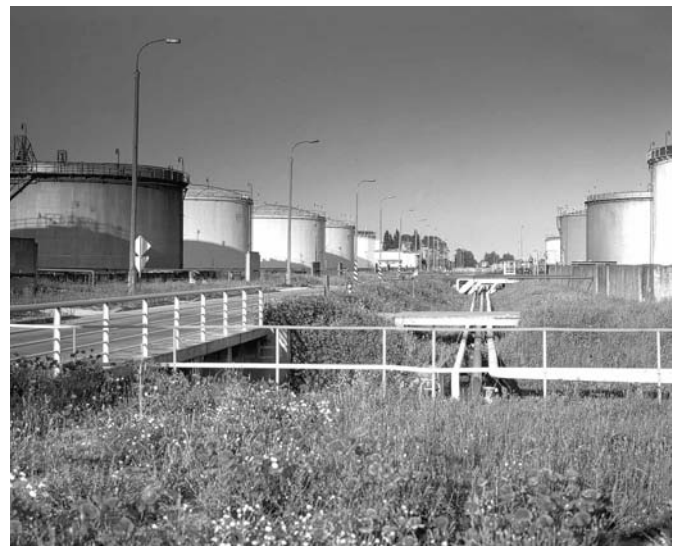
Fig. 23. Typical bulk liquid storage tanks
