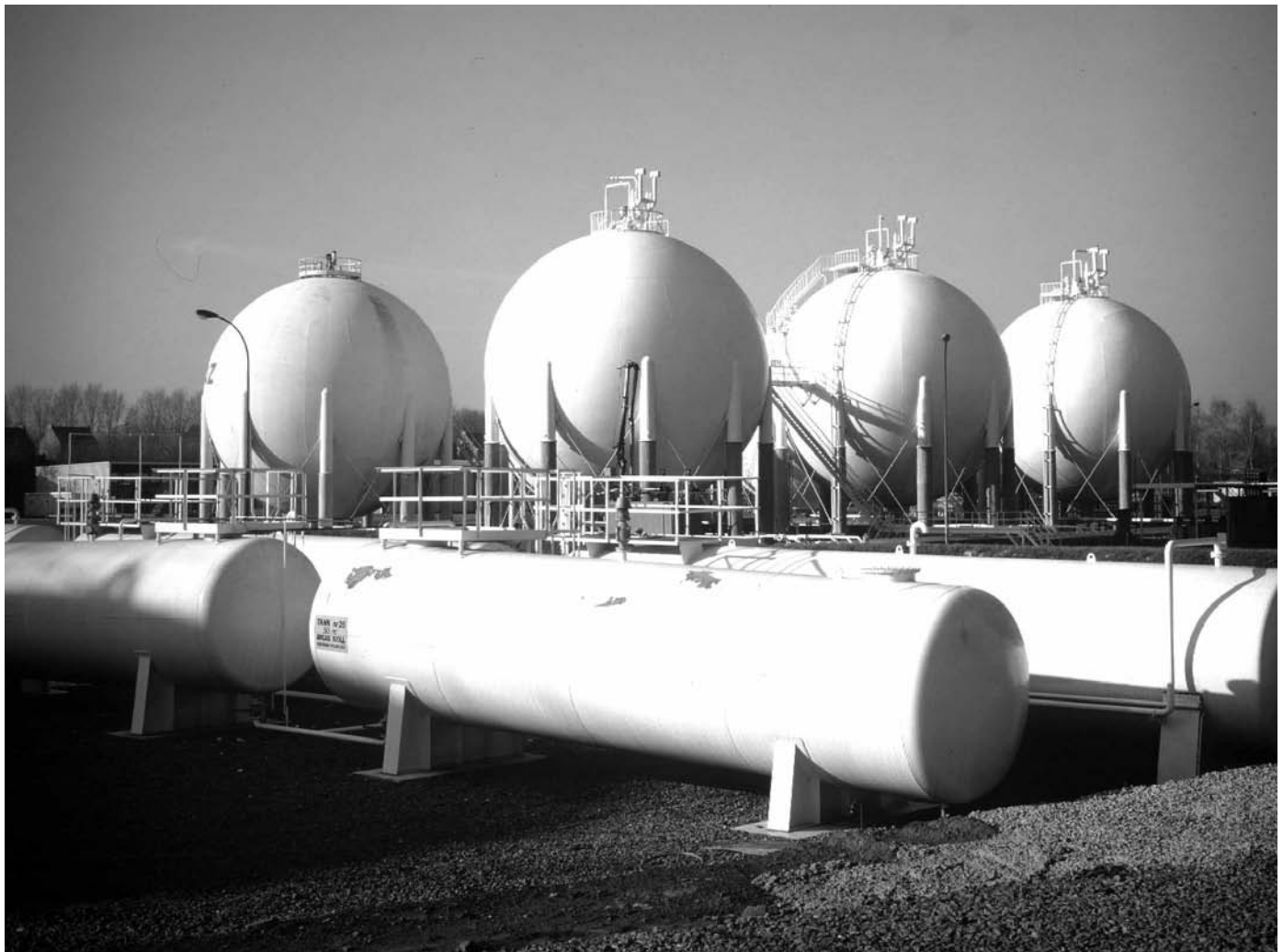
Fig. 31. Pressurized gas storage facility
